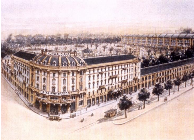
General view of the building
